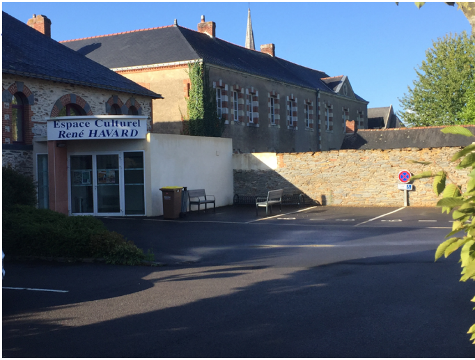
Entrée Route de Guéméné
